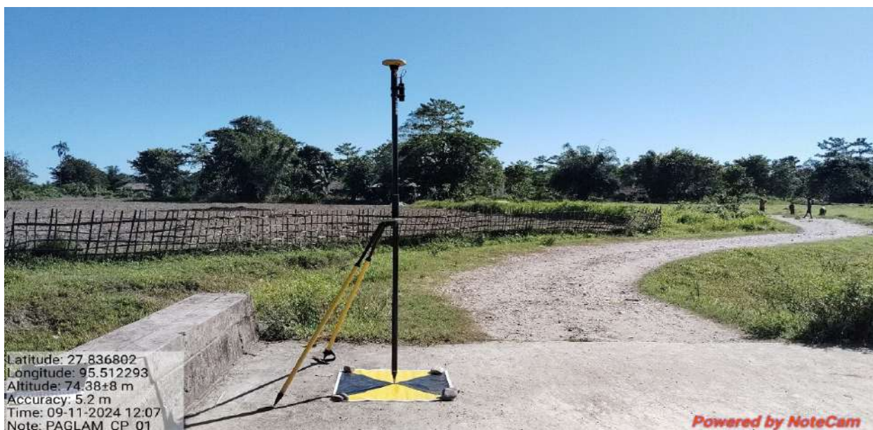
Fig: Drone survey activities at remote village of Lower Dibang Valley district and Shiyomi district, Arunachal Pradesh.
