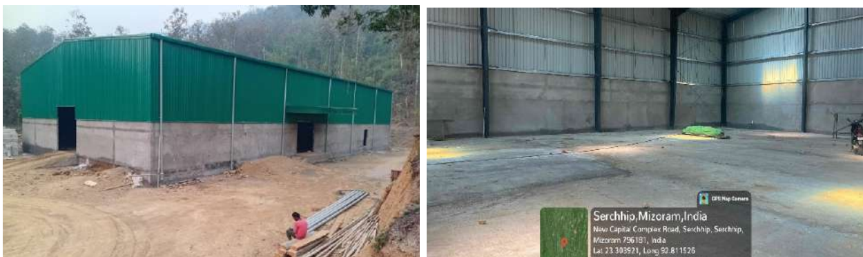
Fig: Construction of Common Facility Centre (CFC) at Serchhip Mizoram
